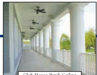
Club House Porch Ceiling
