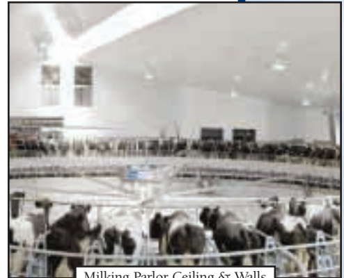
Milking Parlor Ceiling & Walls
