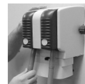
6. Attach short discharge tube on 1 GPM (grey) eductor, then attach longer discharge tube on 3.5 GPM (yellow) eductor.
